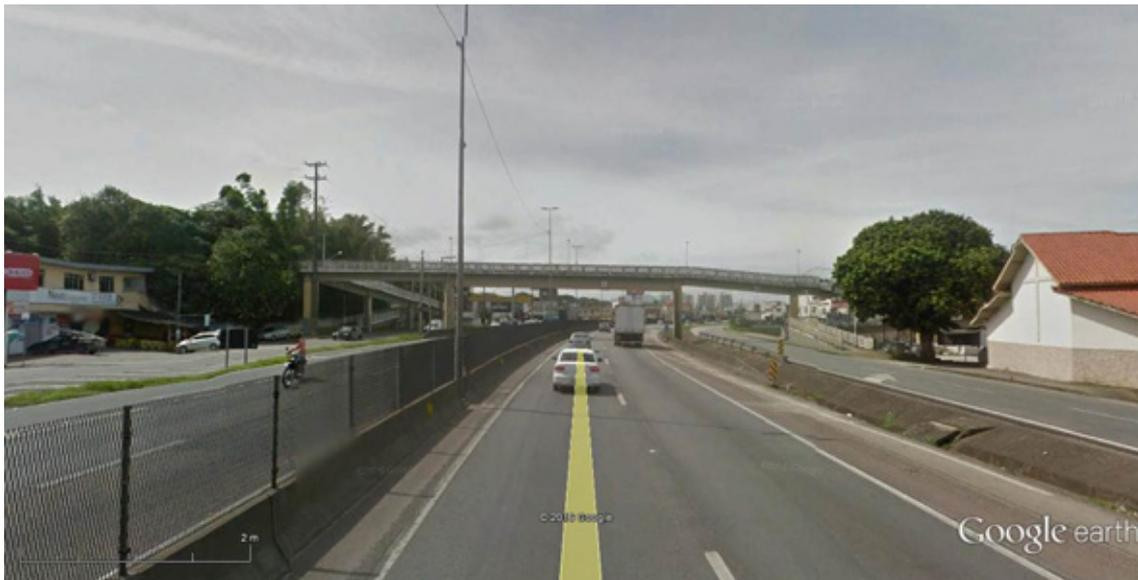
Figure 2 - Example of crossing urban roads with divided lanes and barriers, with only a few transpositions.
